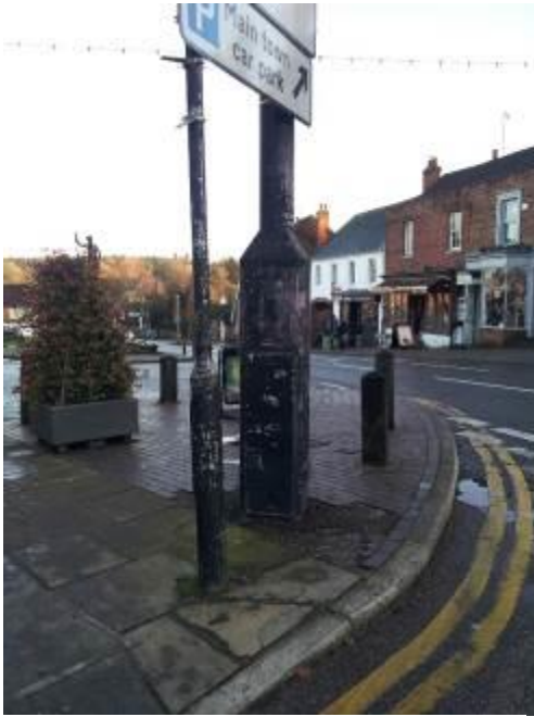
Street furniture in need of maintenance
