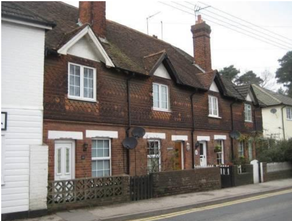
51-55 London Road – shaped tiles, gablets and tall chimneys
