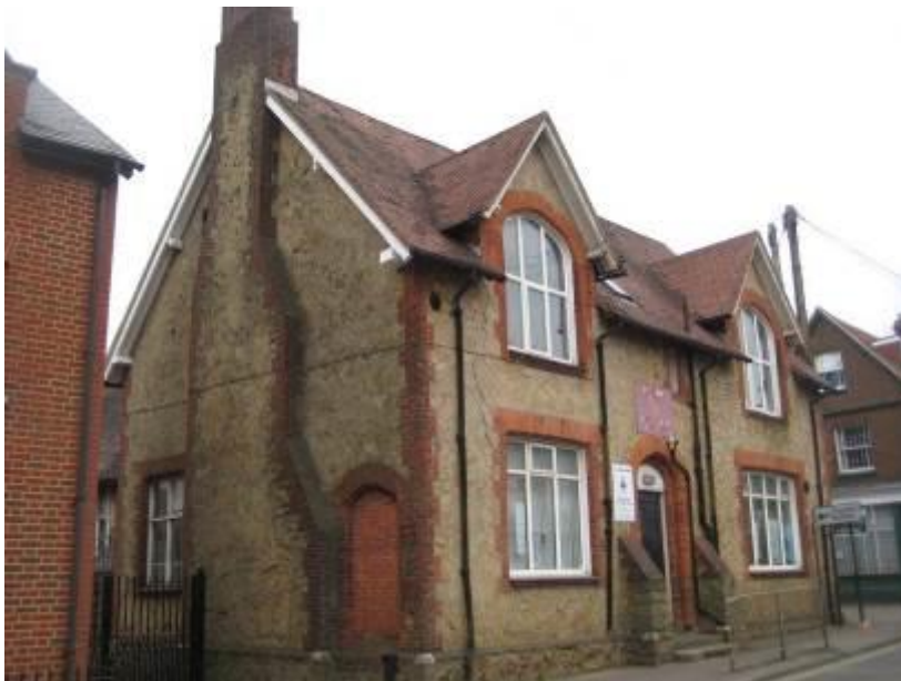
Local sandstone built Drill Hall at corner of Stratton Terrace
