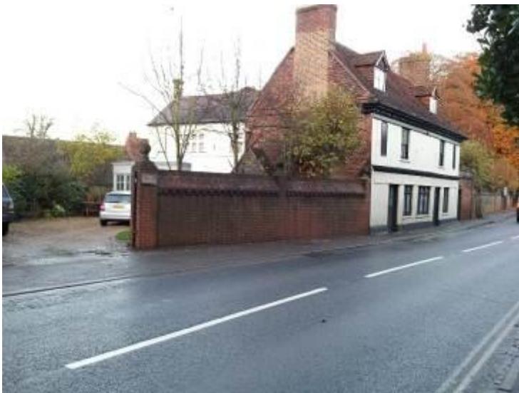
Substantial brick boundary wall at The Old House, Vicarage Hill
